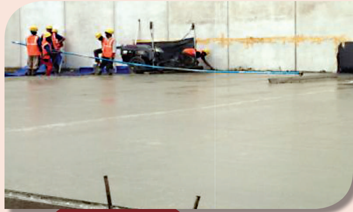
Bump Cutter with the key hole profile
