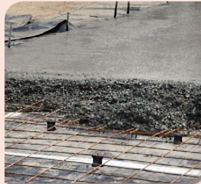
Laying concrete using Steel Bar Reinforcement
