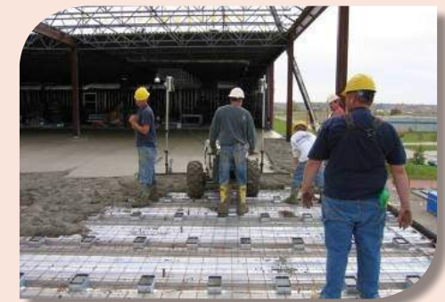
Laying over Metal Deck
