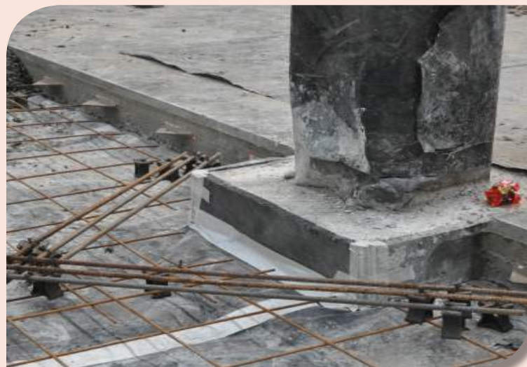
Column Isolation with Auxiliary Reinforcement
