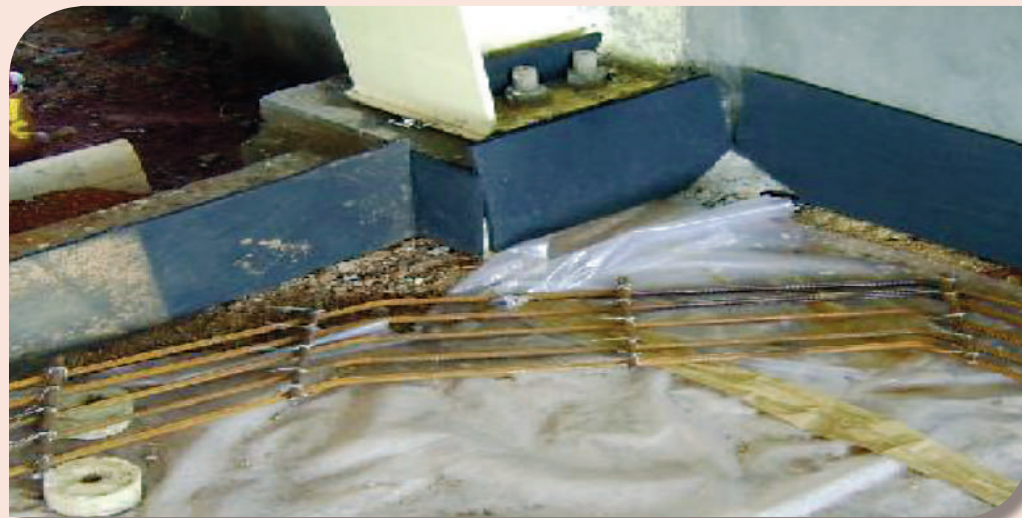
Wall Isolation with Auxiliary Reinforcement.
